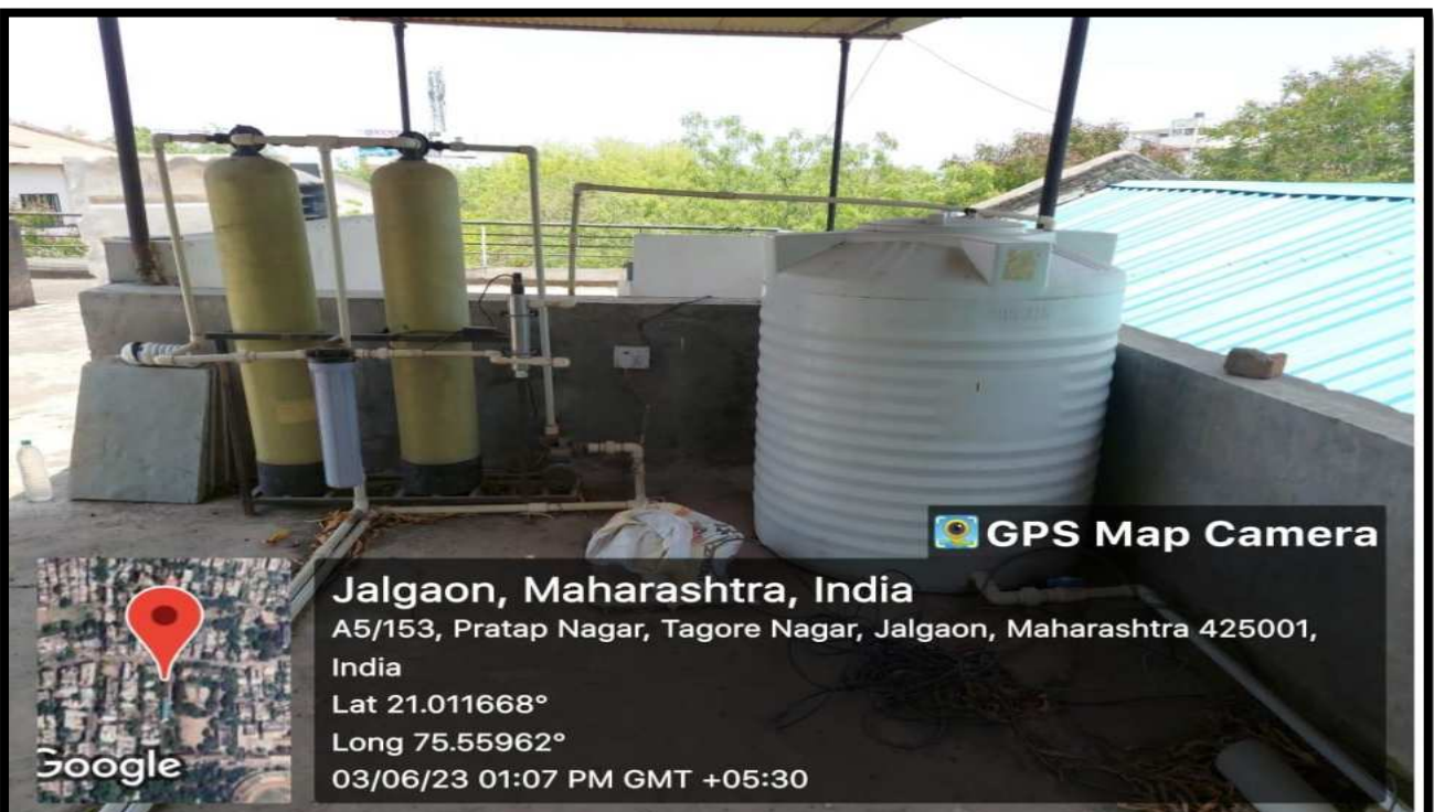
Water Purification RO Plant capacity of 1000 litres.
